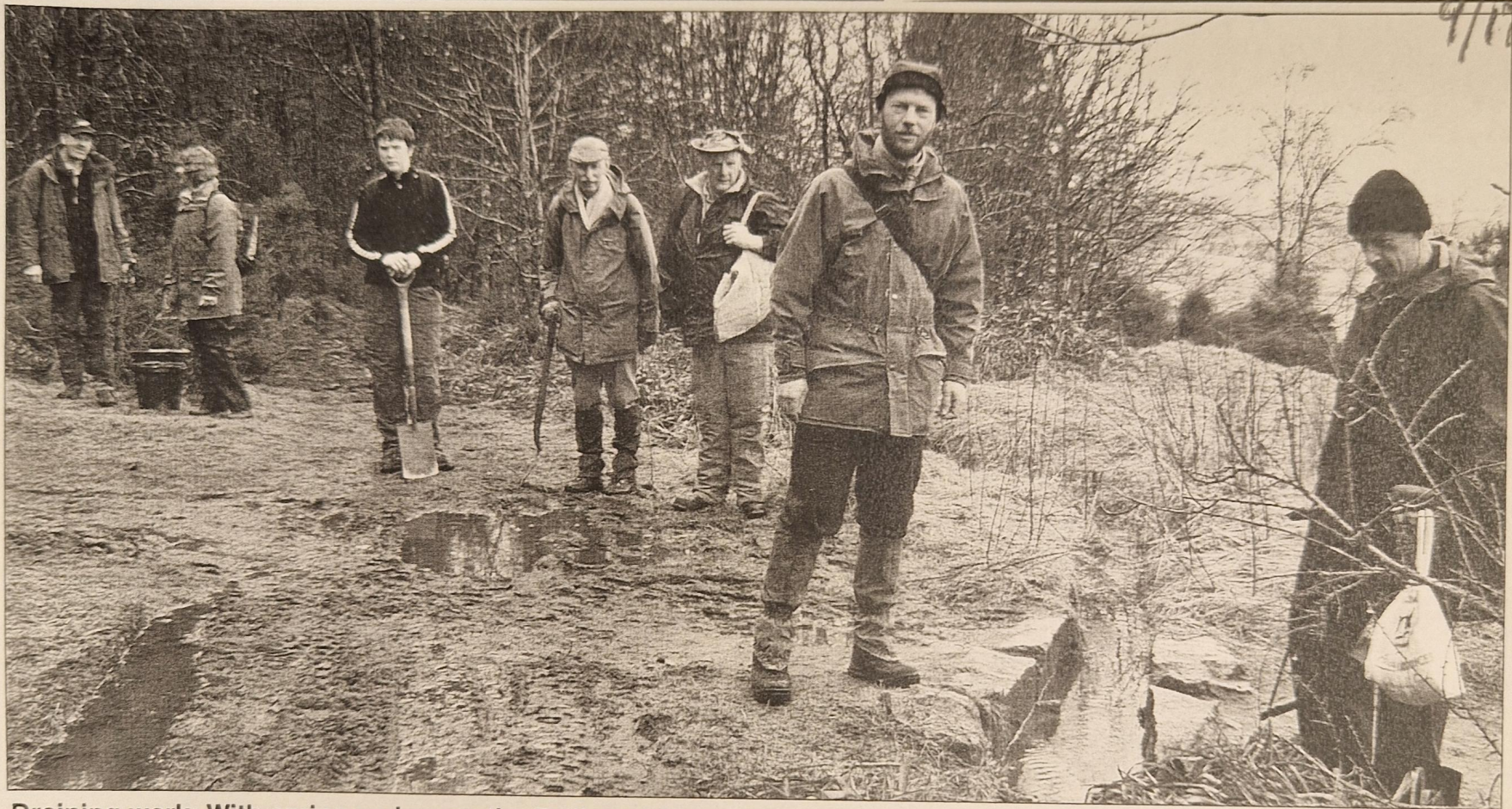
Draining work: With spring underway, the Bailies of Bennachie organise a work party, clearing drains and cutting scrub encroaching on the path from the Rowantree carpark. Photograph by Ellice Milton
