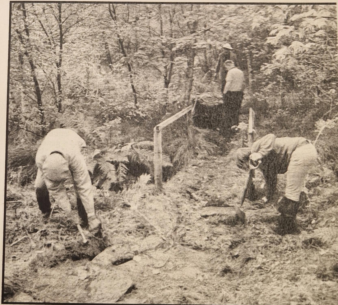
REPAIR JOB: Volunteers at work repairing paths on Bennachie.
