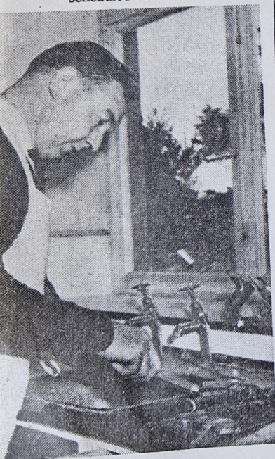
puts the finishing touches to the sink unit in the public-house.
